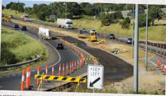
IMPORTANT WORK: The roadworks continue and a plan of the project.
